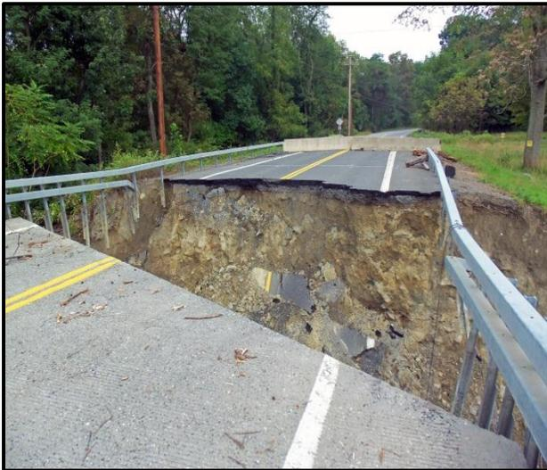
Fluvial erosion along the Moodna Creek contributed to the undermining of portion of the County Route 74/Forge Hill Road bridge in the Town of New Windsor during the tropical storms of 2011.
