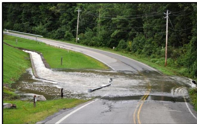
A culvert under Museum Village Road was unable to accommodate high flows resulting from a storm event. Such a scenario is a common cause of ponding and flooding throughout the Moodna Creek Watershed.
