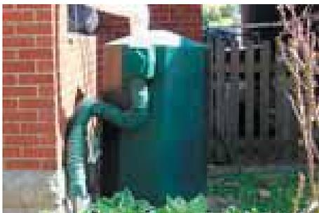
Rain barrels are a tank for temporary storage of rainwater. Stormwater runoff from the roof of a building is diverted through the downspout into a barrel and stored for later use, such as landscaping or cleaning outbuildings.
