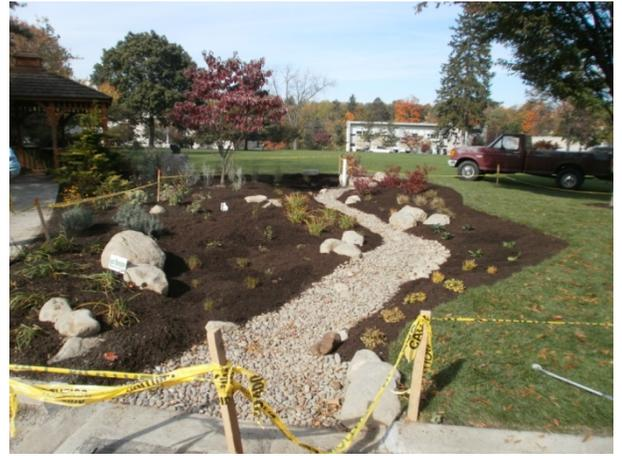
Bioswales are vegetated, mulched, or xeriscaped channels that provide treatment and retention as they move stormwater from one place to another. Vegetated swales slow, infiltrate, and filter stormwater flows. As linear features, vegetated swales are particularly suitable along streets and parking lots.
