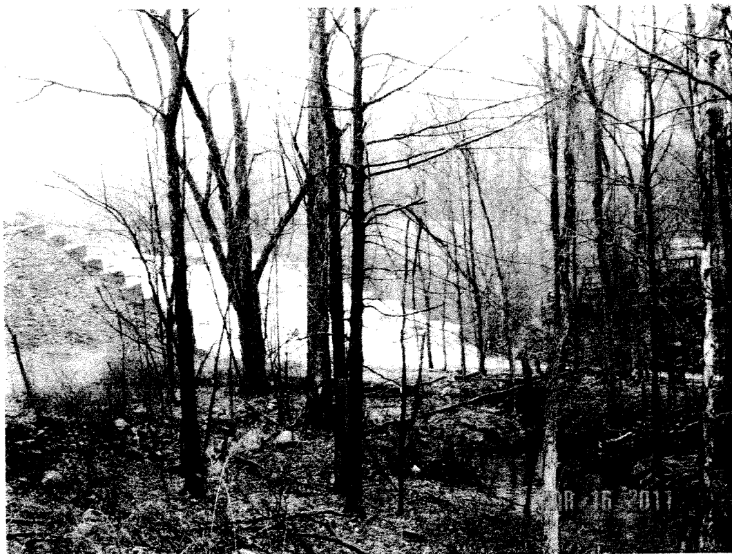
Photo # 2 – Existing woodland near stream at bottom of spillway – area not to be disturbed.
